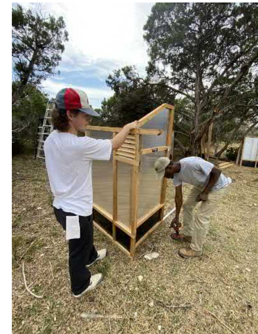
One person can hold panel while the other drives in the screws.
